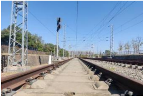
(a) Railway track base
