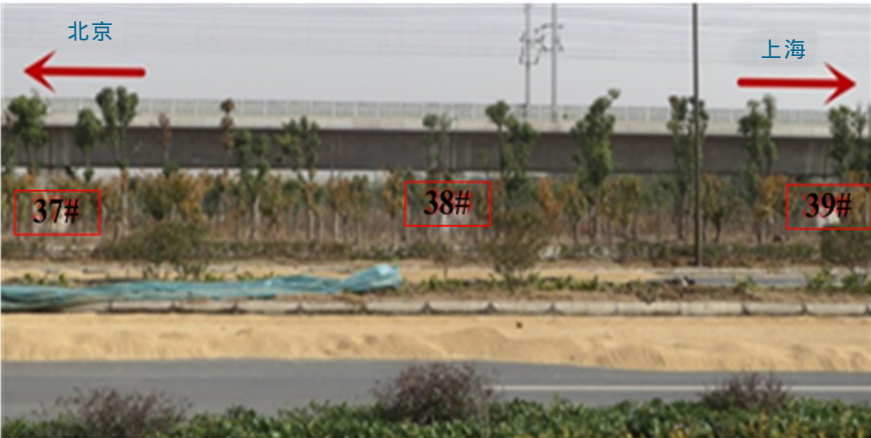
图 1 下穿位置实景 Fig.1 The real scene of the construction location
