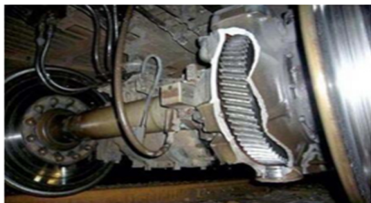
(c) 箱体开裂
