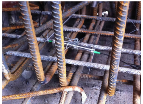
图4 底板传感器S3的固定安装 Fig.4 Fixed mounting of floor sensor S3
