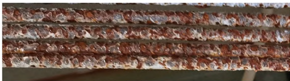
(c) Corrosion time 1 080 h
