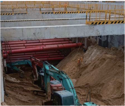
图9 现场土方开挖施工图 Fig. 9 On-site earthwork excavation construction drawing
