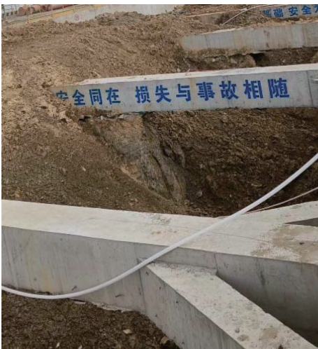
图4 开挖6 m时现场工况 Fig. 4 Site conditions at 6 m of excavation
