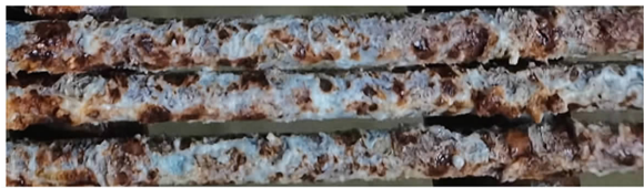
(b) Corrosion time 720 h
