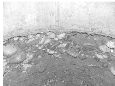
图 3 探坑揭露<2-9-3>地层实况 Fig.3 Geologic situation of layer <2-9-3>
